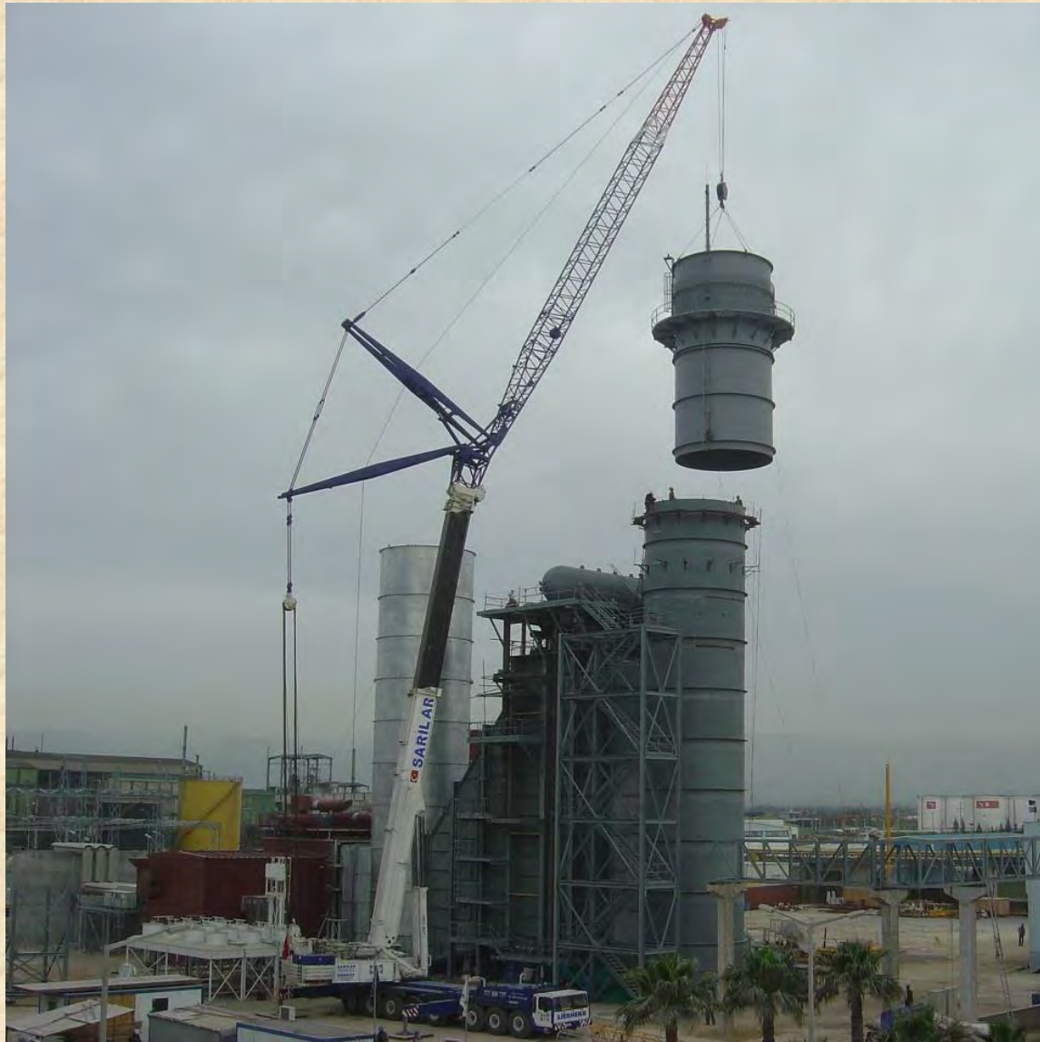
Project: 125 MW Combined Cycle Power Plant for SODA Factory - Phase I, Mersin, TURKEY Client: Nooter/Eriksen Inc. Scope: Exhaust Stack, Stair Tower, Ladders, Platforms
